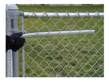
Insert the patented locking strip horizontally into the top section of the 2nd diamond down from the top of your chain link fence.
