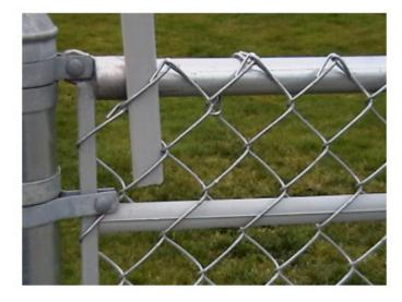
Insert the slats vertically until the patented notch snaps itself into the locking strip.
