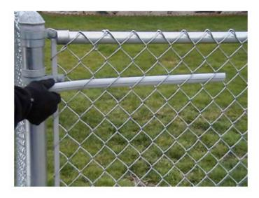
Insert the patented locking strip horizontally into the top section of the 2nd diamond down from the top of your chain link fence.
